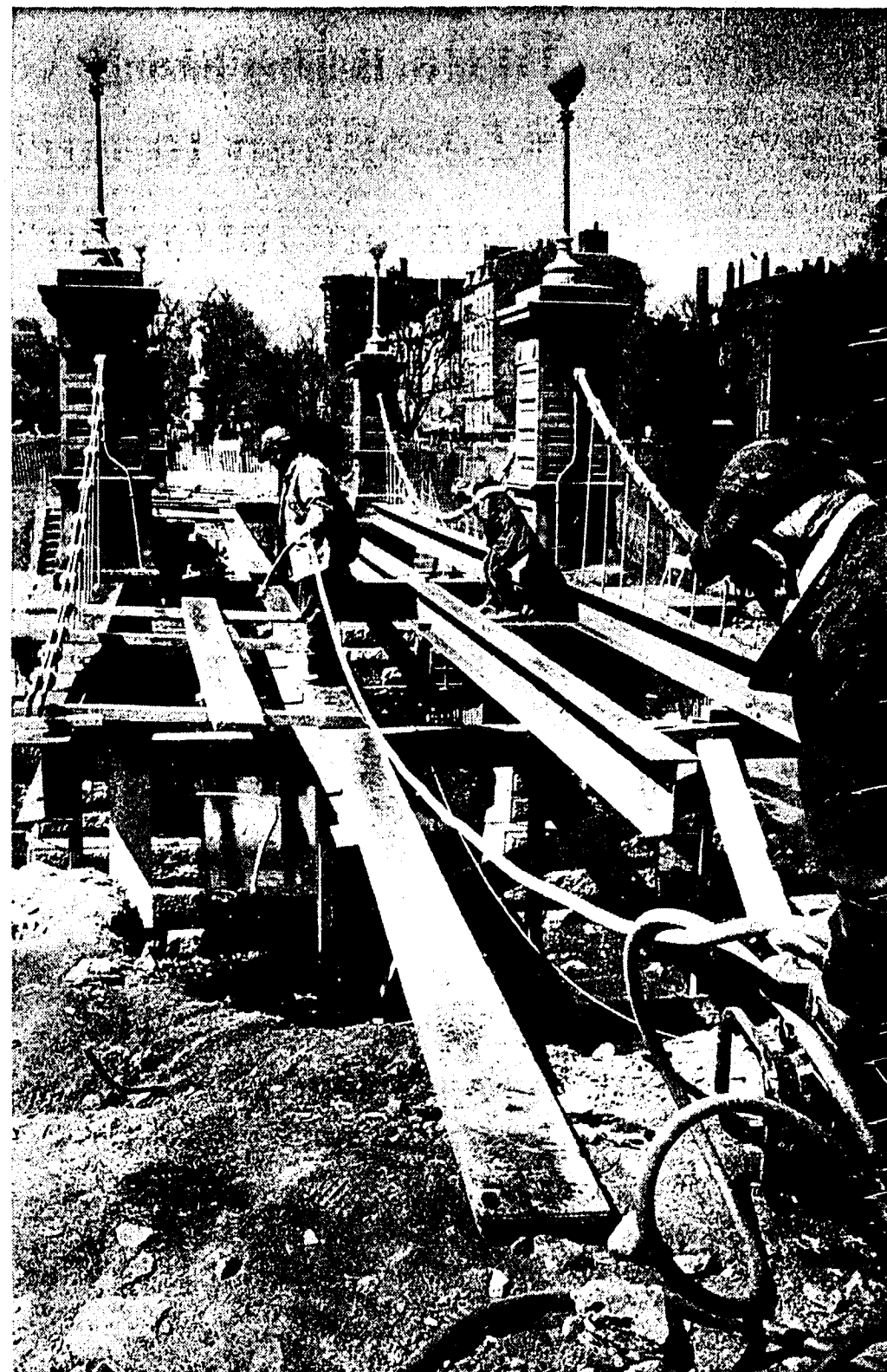
Bridge over pond in Boston's Public Garden is stripped of its surface as workmen undertake task of re-
